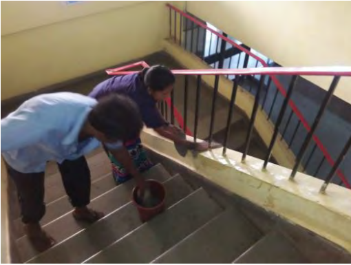
Fig 4.1.10 Aisles and Stairway
