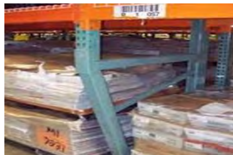
Fig4.1.19 Storage rack beam damage
